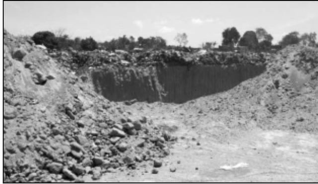
Photograph 15. Special Trench at a Controlled Area of a Landfill for Treated Waste From Microwave Treatment
