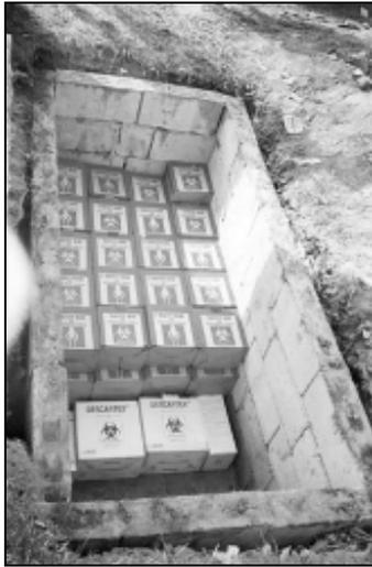
Photograph 17. Safety Boxes Being Encased in a Concrete Vault at a Cemetery
